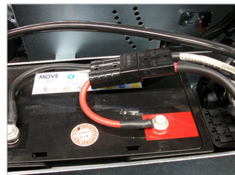
Fig. 46: Main cable battery
